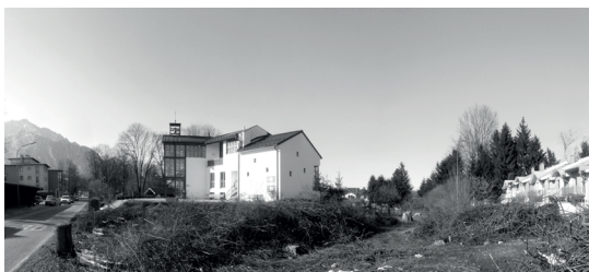
Respecting the local Topography and Integration of the existing parish community building
