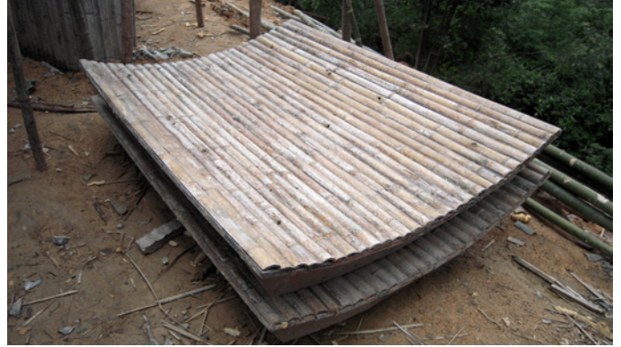
Bamboo Formworks
