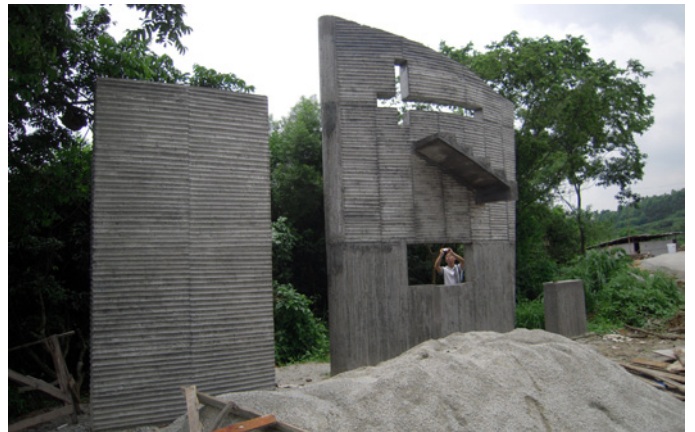
Concrete Wall Mock-up
